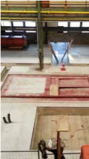
Fundamentarbeiten beendet Foundation work finished
